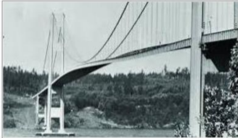
Fig. 1: The carriage way of the bridge is excited to torsional vibration 1
